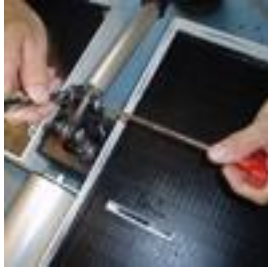
Hinge bolt removal
